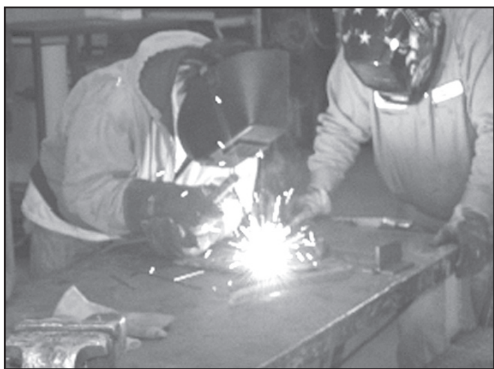
Clayton Appelhans was welding while Tanner Corder watched at the Northwest Kansas Technical College Ag Mechanics, Farm Power & Machinery, and Electrical Contest held in Goodland last week.
