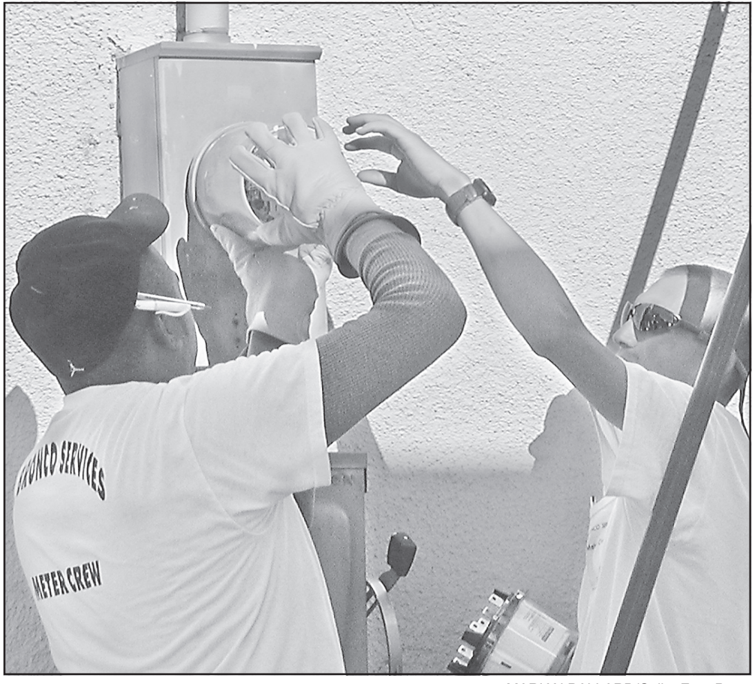
MARIAN BALLARD/Colby Free Press The strangers in bright T-shirts seen in alleys and backyards around town include Bob Howard of Texarkana, Texas, (right) and Alonso Noriega of Dallas, who were busy changing the electric meter at the Colby Free Press office this morning. Employees of contractor U.S. Bronco Service out of Ohio, they say it's cooler in Texas this summer than here.
