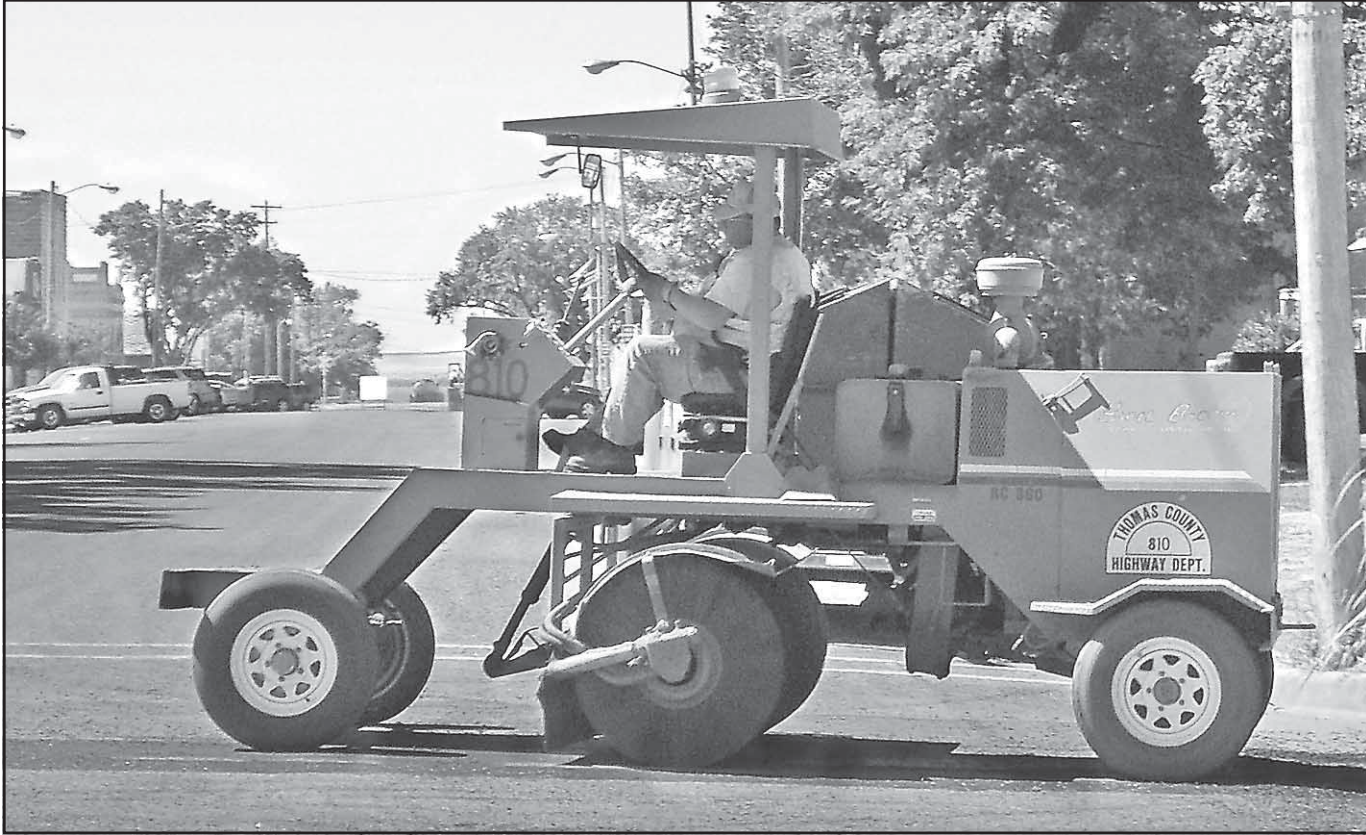
HEATHER ALWIN/Colby Free Press This week, County crews were out sealing a stretch of Old 24 between Brewster and Levant (above and left). Thomas County road workers were sealing streets in Brewster in 100+ degree weather last Friday. After the streets were oiled and crews press a layer of rock into the sticky goo, Darrin Bell, a highway department employee, swept off the loose gravel (above).
