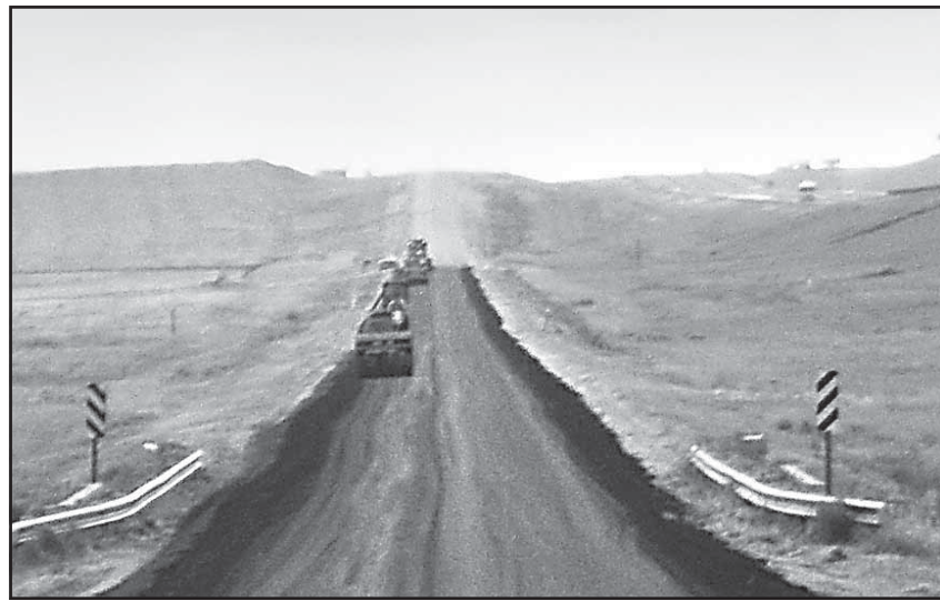
HEATHER ALWIN/Colby Free Press This week, County crews were out sealing a stretch of Old 24 between Brewster and Levant (above and left). Thomas County road workers were sealing streets in Brewster in 100+ degree weather last Friday. After the streets were oiled and crews press a layer of rock into the sticky goo, Darrin Bell, a highway department employee, swept off the loose gravel (above).
