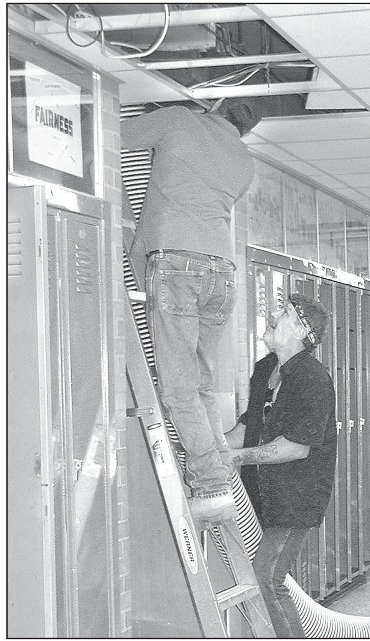
Rusty Depe (above) started a motor which powers a large vacuum system being used to clean duct work at Colby
