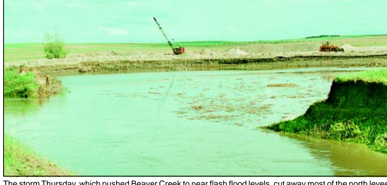
The storm Thursday, which pushed Beaver Creek to near flash flood levels, cut away most of the north levee at Allied Inc.'s gravel pit north of Goodland. Officials at the firm's Hays office said they are pumping the water out, but they are not sure when the pit will be back in operation.
