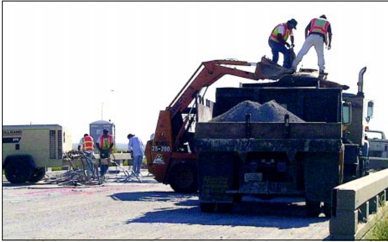
Workers for Koss Construction (above) are ripping out the old surface and preparing the ground for new paving as part of the resurfacing process of the eastbound lanes of I-70. Other crews are working on the deck of the I-70 overpass of Business U.S. 24 and two other bridges in the eastbound lanes.
