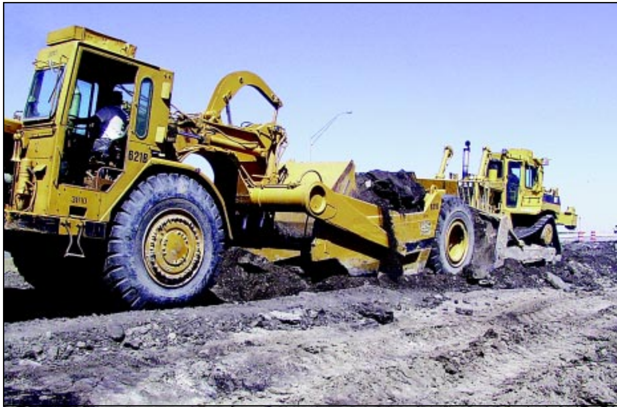
Workers for Koss Construction (above) are ripping out the old surface and preparing the ground for new paving as part of the resurfacing process of the eastbound lanes of I-70. Other crews are working on the deck of the I-70 overpass of Business U.S. 24 and two other bridges in the eastbound lanes.
