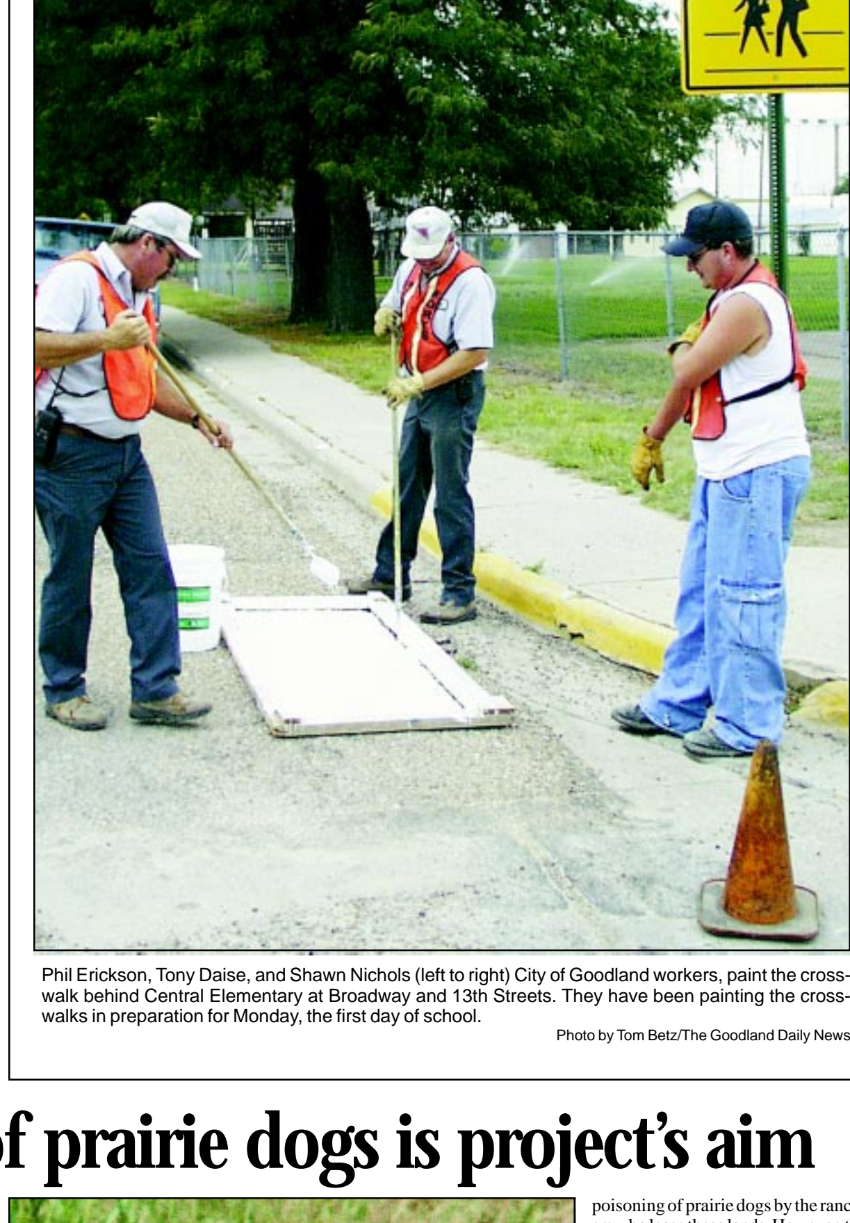
Phil Erickson, Tony Daise, and Shawn Nichols (left to right) City of Goodland workers, paint the crosswalk behind Central Elementary at Broadway and 13th Streets. They have been painting the crosswalks in preparation for Monday, the first day of school.
