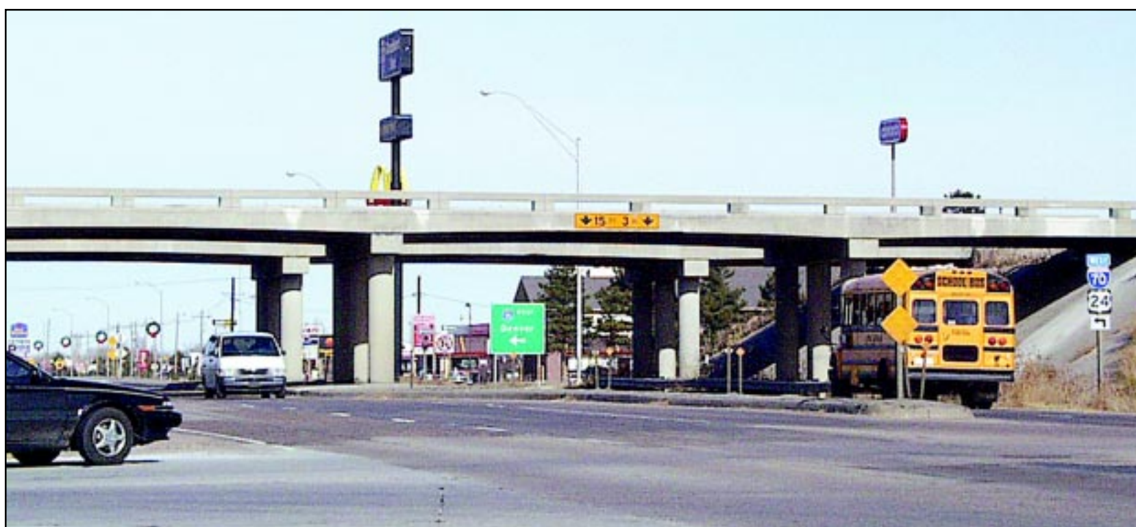
When spring arrives, drivers will find a cone zone to negotiate as the reconstruction of K-27 from Broadcast Plaza north to Business U.S. 24. Kansas Department of Transportation and the City of Goodland begin. Photo by Janet Craft / The Goodland Daily News
