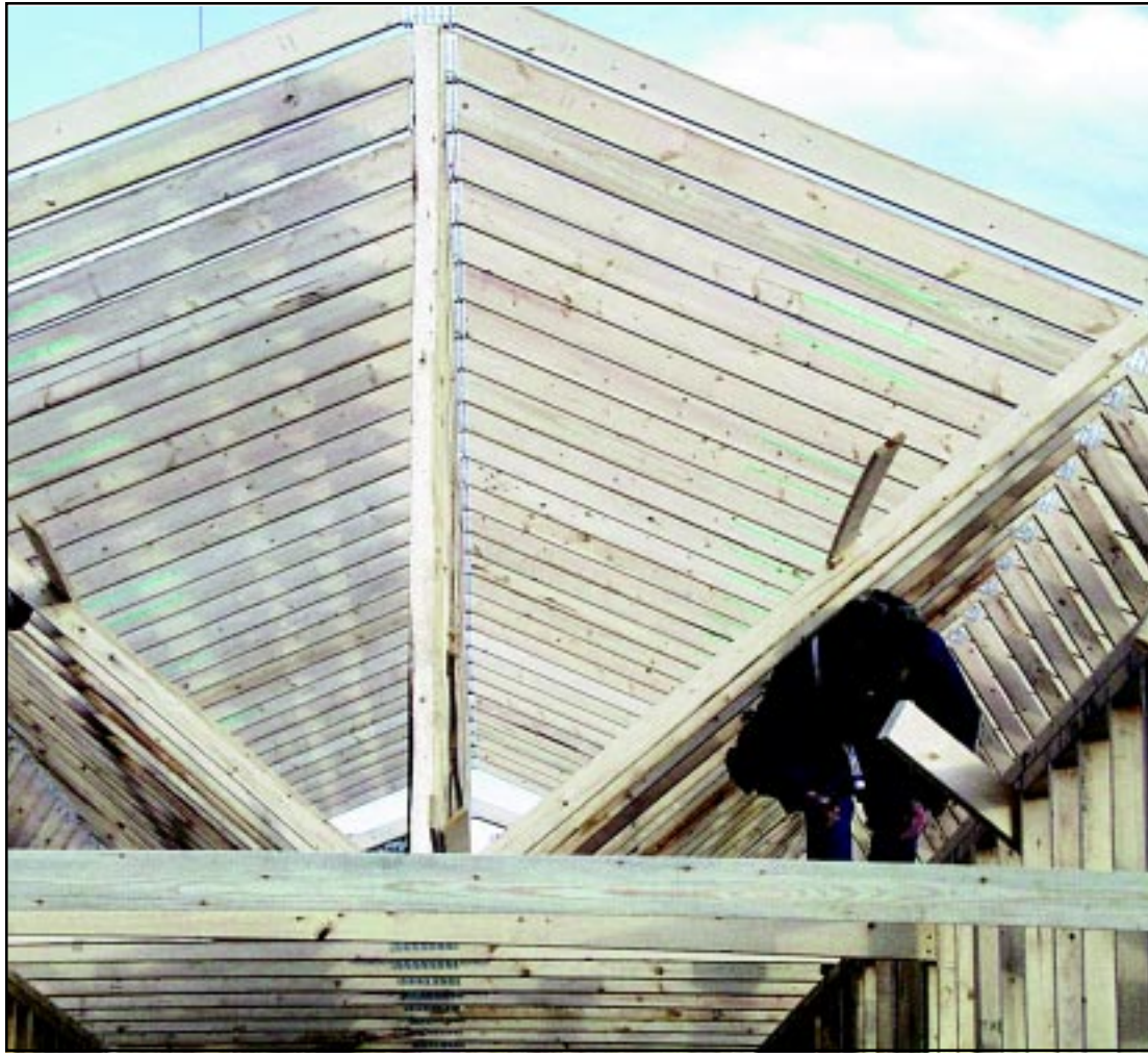
Framing crew members worked at hammering trusses in place for the roof of the Wheat Ridge Acres Assisted Living Center on west 8th Street on Wednesday. Photo by Janet Craft/The Goodland Daily News
