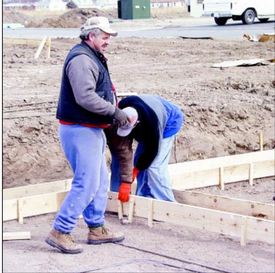
Dave Hutchison, contractor, (front) looked over the concrete forms for a duplex to be built west of Wheat Ridge Acres on Tuesday, while Heath Hutchison held a board for Beau Hodges (partially hidden) to nail in place. Beau Hodges (right) nailed a board in place on the concrete forms for the foundation of the duplex.
