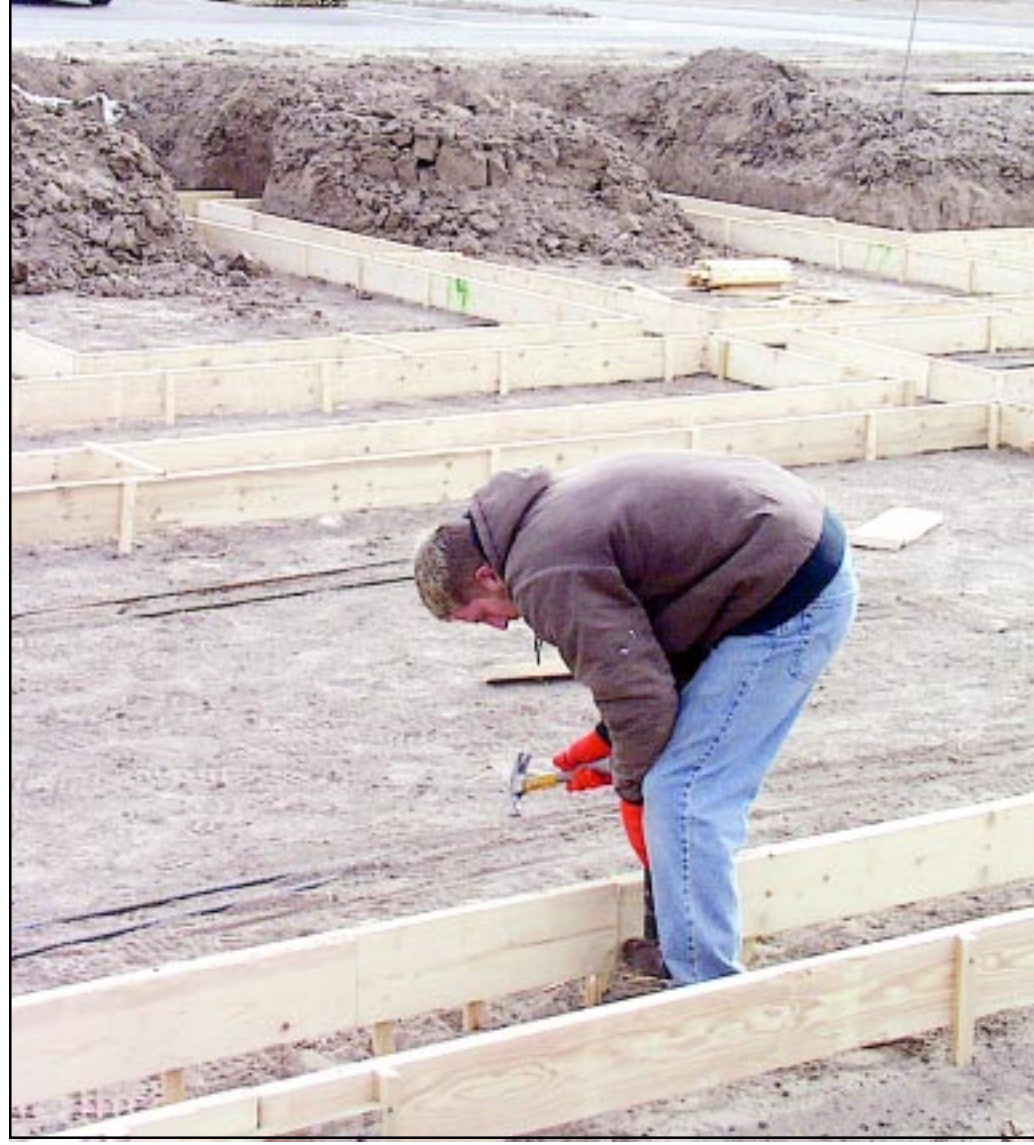
Dave Hutchison, contractor, (front) looked over the concrete forms for a duplex to be built west of Wheat Ridge Acres on Tuesday, while Heath Hutchison held a board for Beau Hodges (partially hidden) to nail in place. Beau Hodges (right) nailed a board in place on the concrete forms for the foundation of the duplex.
