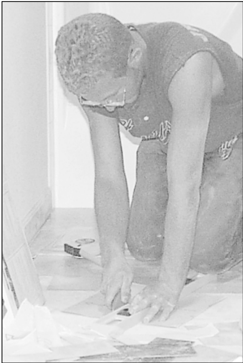
Carpentry students in the 11-month program at the Northwest Kansas Technical School continue work on the three-bedroom home they are building on the school campus. Brandon Pfannenstiel, Hays, cut a linoleum tile to be laid in the bathroom. The house is scheduled to be complete around July 9, when an open house will be held.
