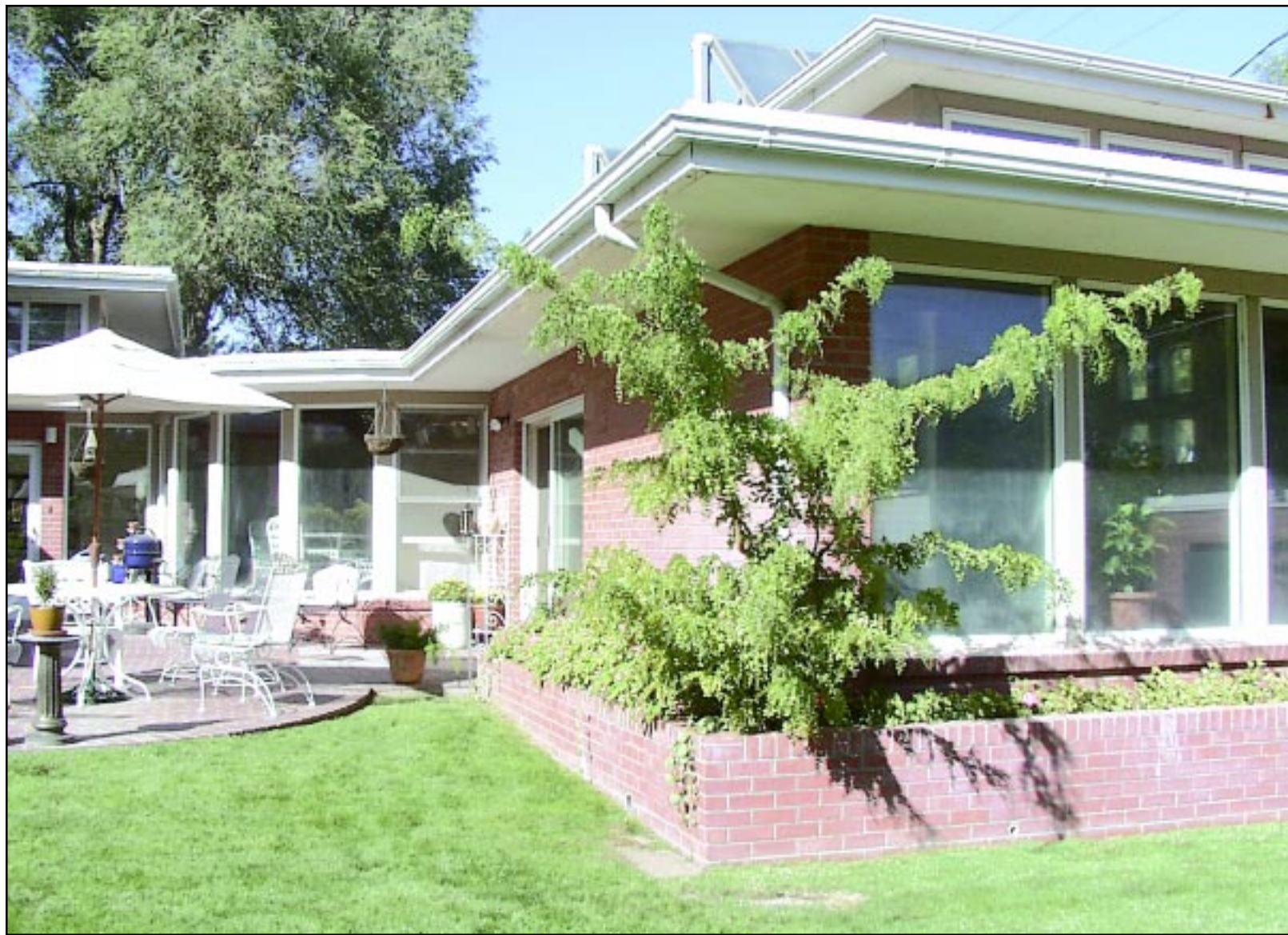
When Russell Withers and his fiancée Carol McClure decided to renovate their home at 525 Main Ave., they tracked down the architect who designed this addition in 1983. They wanted to preserve the historical
