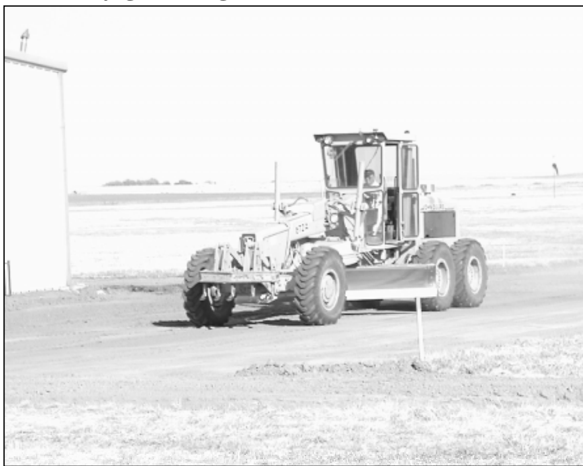
Wilbur Tiede did dirt work on an extension to the taxiway at the Goodland airport Thursday afternoon. Tiede will lay out the dirt for the taxiway, but the city hasn't found a company to do the asphalt work yet. Photo by Dana Sulsberger/The Goodland Daily News
