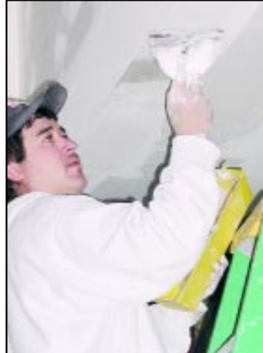
Efrain Rascon applied plaster to a ceiling in the fitness center.
