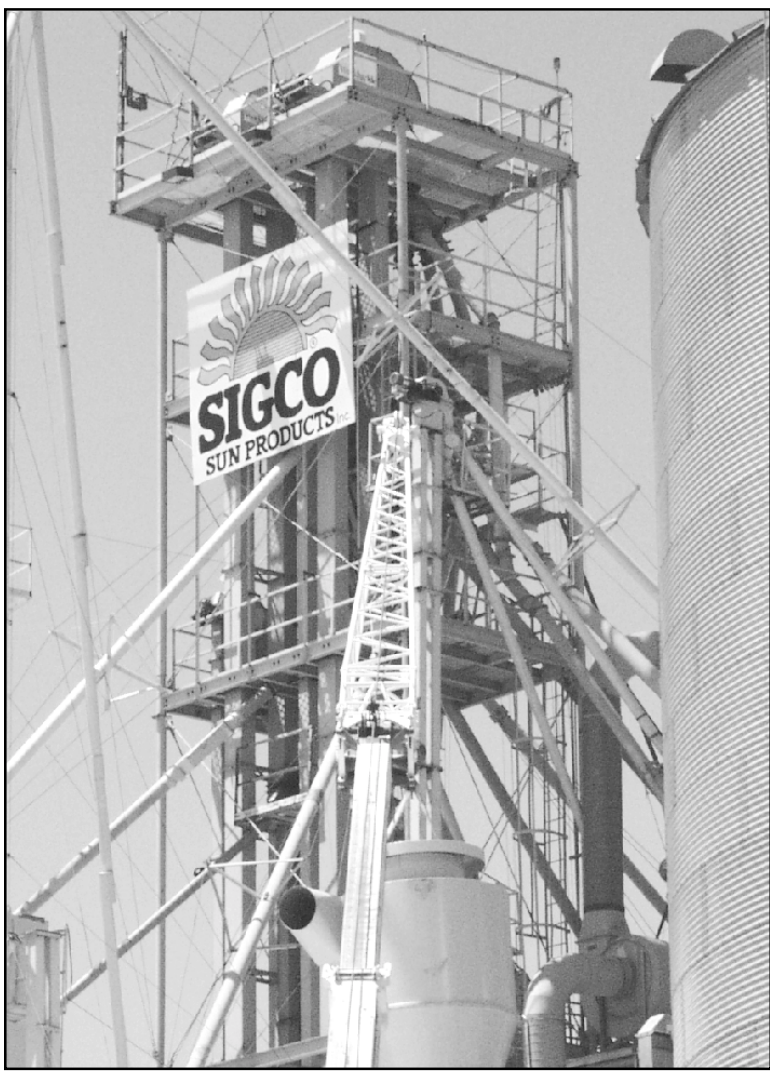
Workers at Sigco Sun Products installed new cyclones Friday. They should provide employees with cleaner air with less dust. The cyclones separate dirt from seeds and keep dust out of the factory, said John Bontjes, plant manager.
