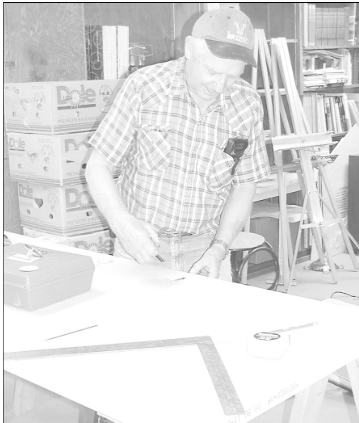
Rich Whitmore put a doorknob in the door he was installing at the Carnegie Arts Center on Thursday. He had help from Duane Hanke — both are on the board at center. The door and the rental tools to install it were donated by Rasure Lumber.
