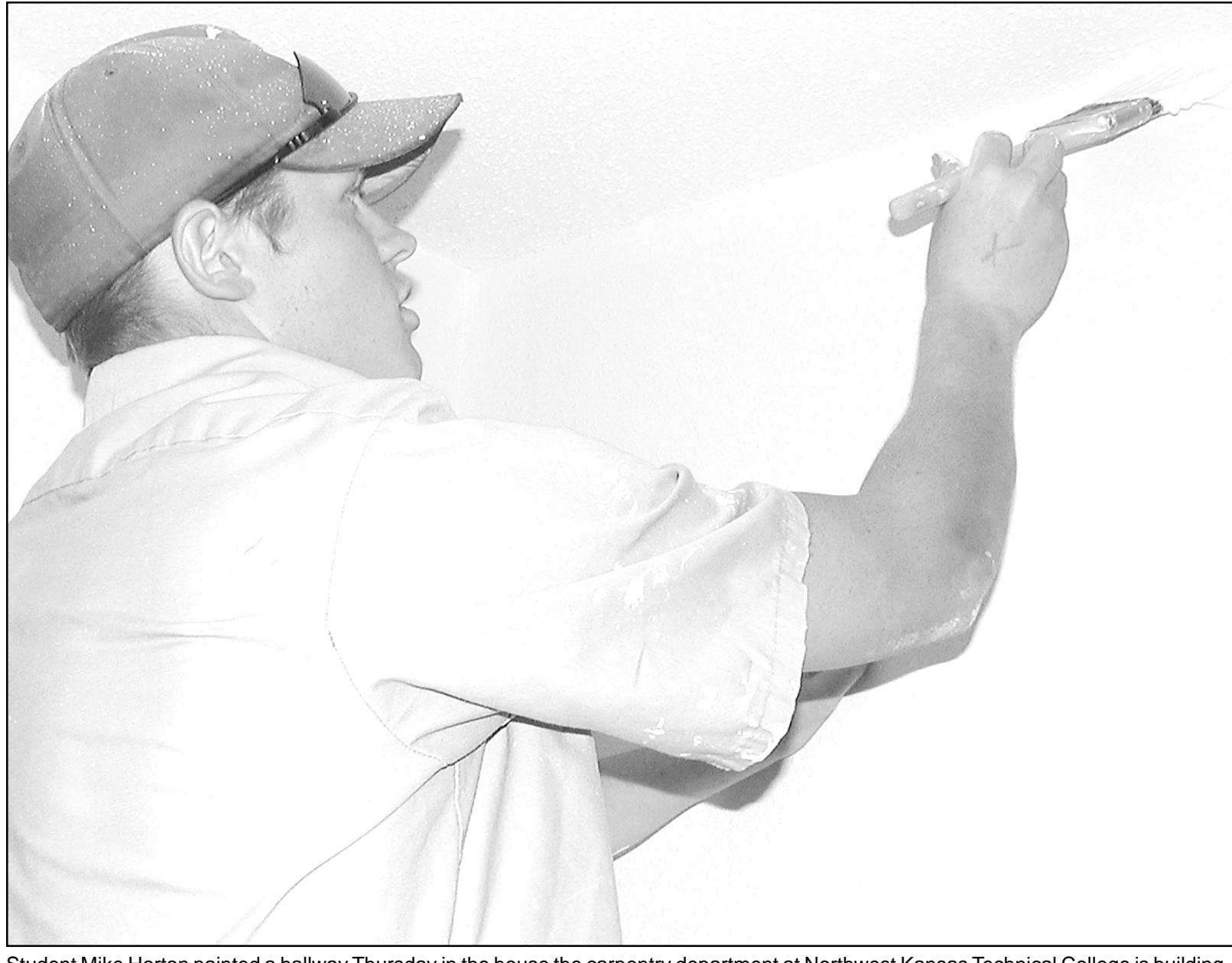
Student Mike Horton painted a hallway Thursday in the house the carpentry department at Northwest Kansas Technical College is building. Photo by Doug Stephens/The Goodland Daily News
