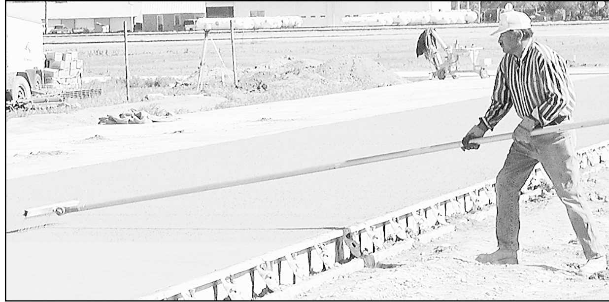
A worker from Ritchie Paving, the contractor working on the road construction in Goodland, lined freshly poured concrete on Wyoming near Business U.S. 24 on Friday morning. Photo by Doug Stephens/The Goodland Daily News
