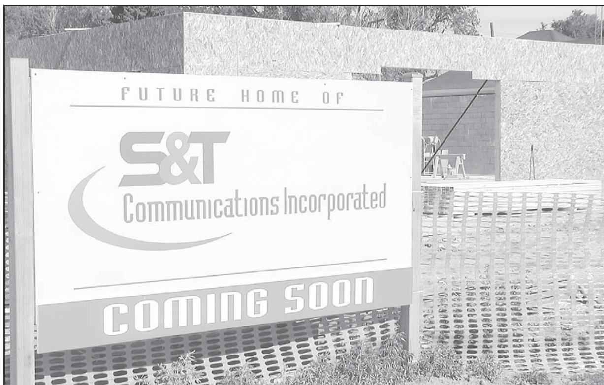
A sign the Brewster-based S&T telephone company put outside the Goodland office, which is currently being built on Main Ave. The office should be done this fall.
