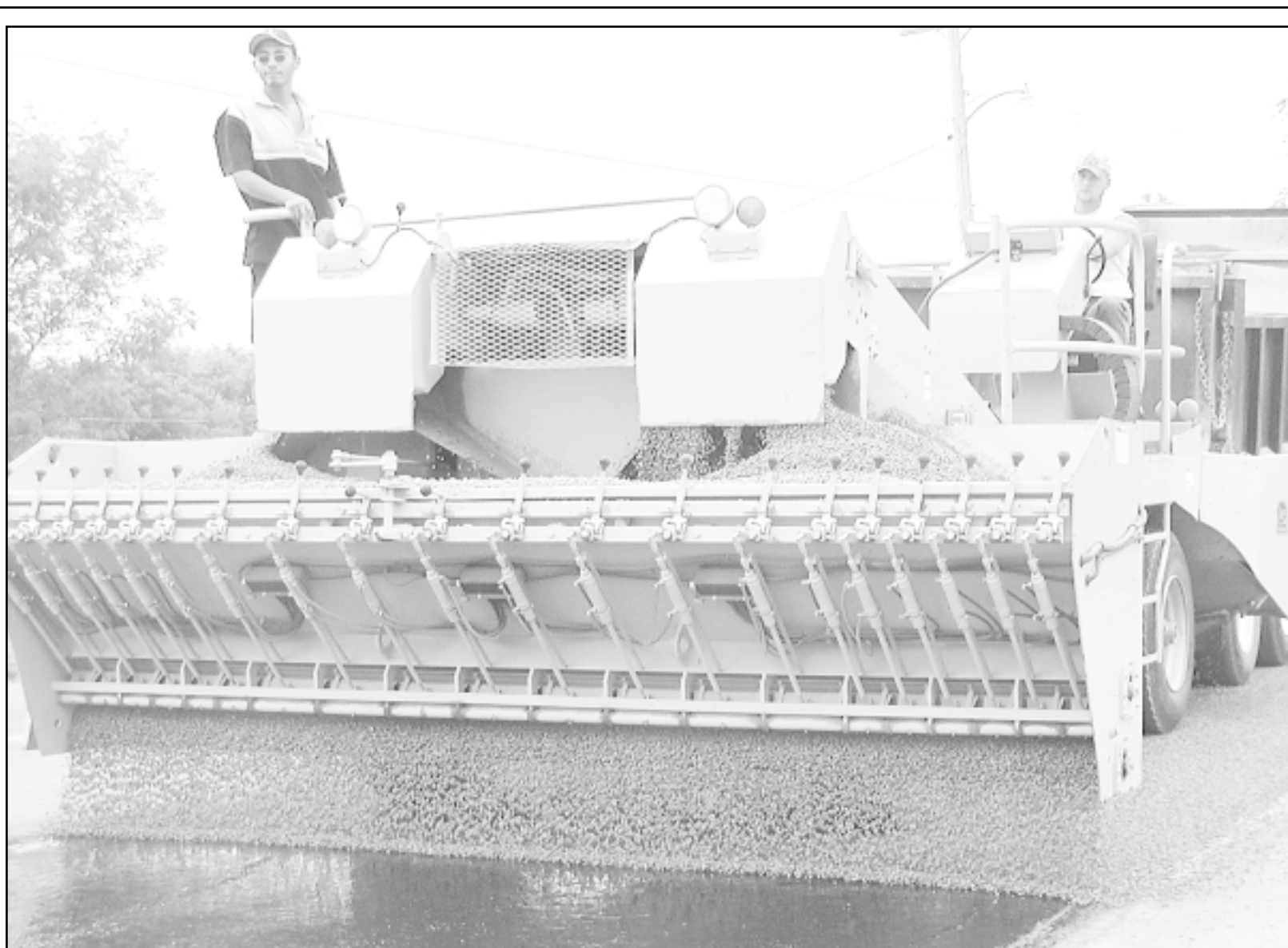
Workers with B&H Paving, out of Scott City, stood on a machine that was spreading crushed rock on Goodland's streets this morning. An oil sprayed on the road helped keep the rock in place. The process is called "chip sealing" and the city uses it to maintain streets. A third of the streets in Goodland will be sealed in the next week. Photos by Rachel Miscall/The Goodland Daily News
