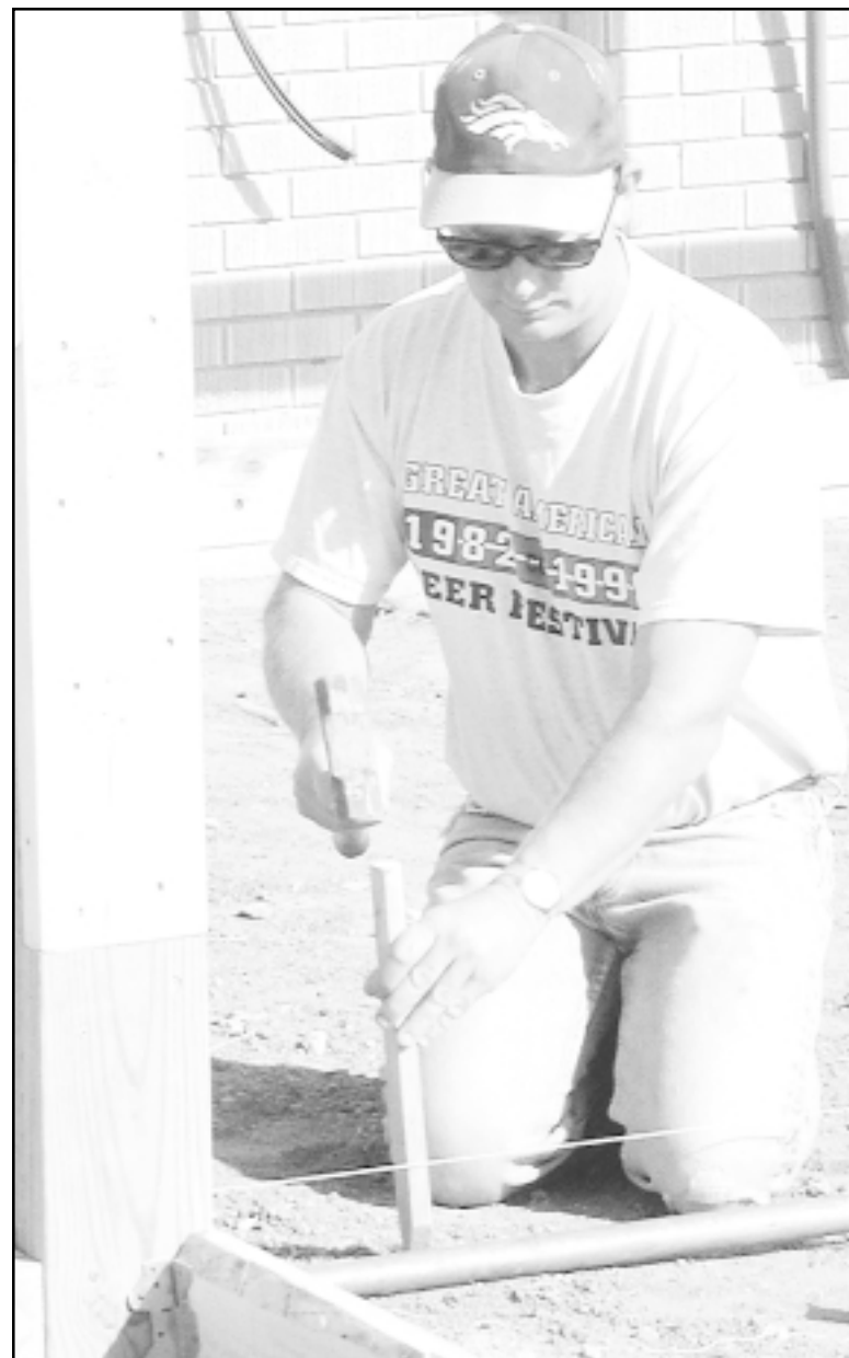
John Morton of Morton Construction hammered in stakes behind the Prints and the Paper at 12th Street and Broadway. The owner of the building, Rod Cooper, is adding storage units to the property. Photo by Doug Stephens/The Goodland Daily News
