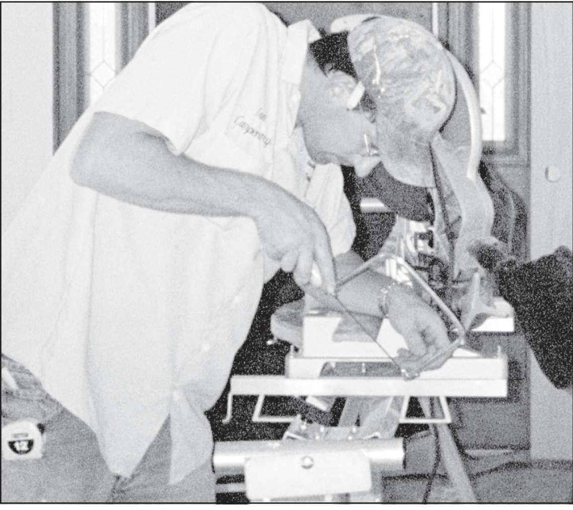
Carpentry student Ian Kohart used a coping saw to make some fine cuts in molding he was installing in the house the technical college students have been finishing for the open house on Sunday. Photo by Bill Wagoner/The Goodland Star-News
