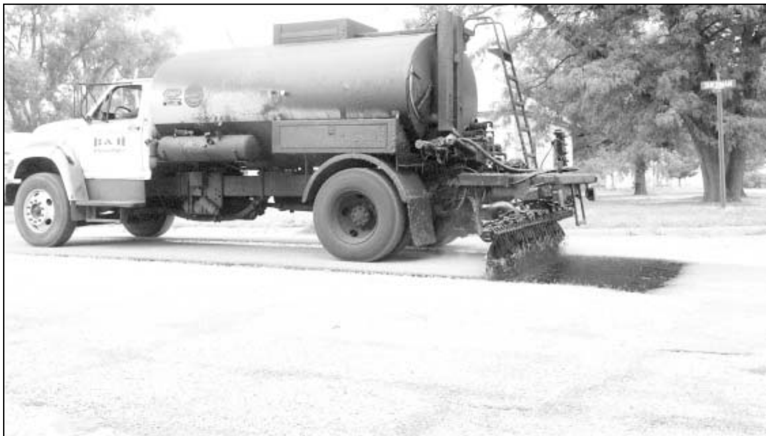
Workers with B&H Paving of Scott City laid down oil and sand to seal Sherman Avenue from Sixth to Ninth on Monday morning as a part of the repaving contract around town. Photos by Shannon Davidson/The Goodland Star-News
