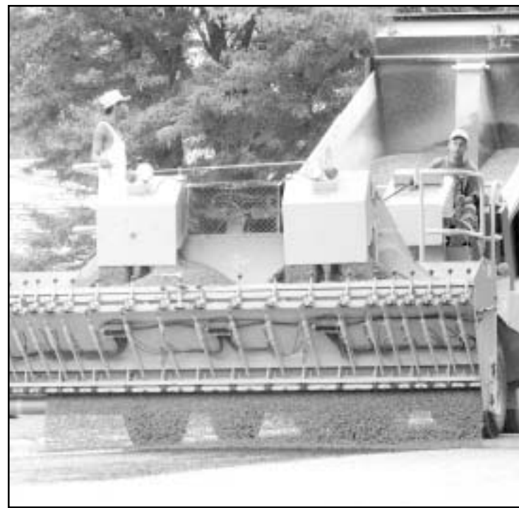
Workers with B&H Paving of Scott City laid down oil and sand to seal Sherman Avenue from Sixth to Ninth on Monday morning as a part of the repaving contract around town. Photos by Shannon Davidson/The Goodland Star-News
