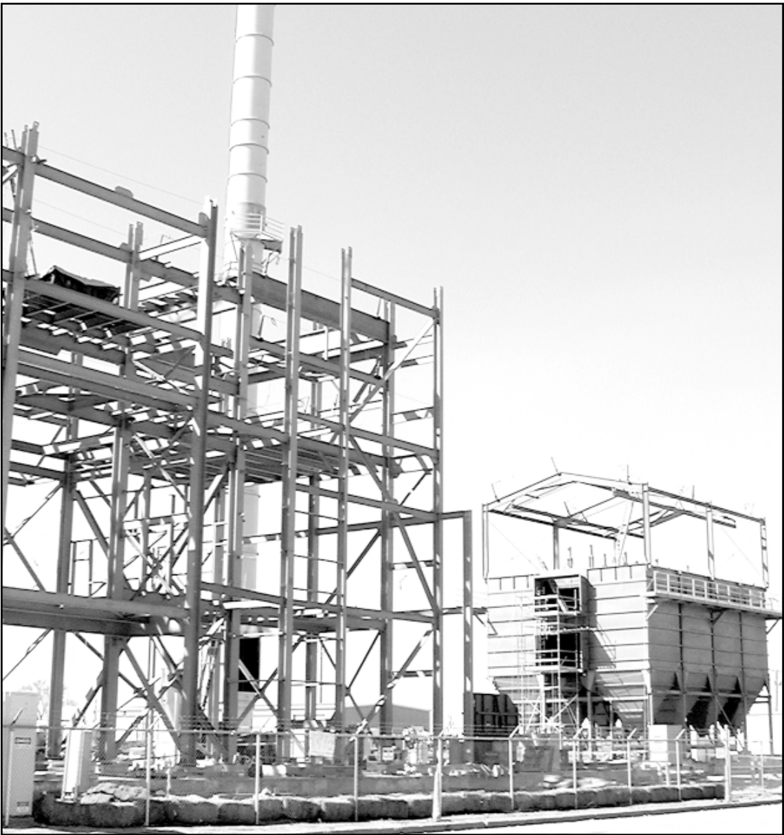
The exhaust stack is up at the new coal-fired power plant at the corner of Second and Oak in Lamar, Colo. The coal bunkers (right) and most of the major pieces are in place and the steel framework has been erected. The project will convert the 1970 city power plant from natural gas to coal with an increase from 25 mega watts to 38 megawatts, serving seven area towns.
