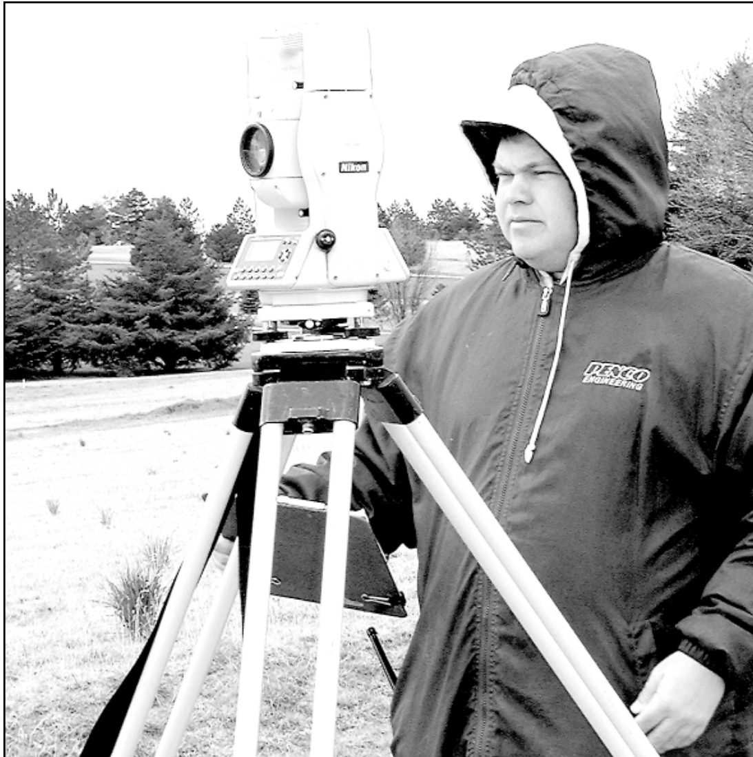
Chat Olmstead of Penco Engineering from Plainville and his partner, Chris Byer, braved chilly winds last Tuesday to complete some survey work on the section of County Road 16 near Sugar Hills Golf Club. Paving the one-mile section is part of the joint city-county road program that includes 17th Street, Caldwell Avenue, Eight Street west of town and old U.S. 24 across the county. Photo by Tom Betz/The Goodland Star-News
