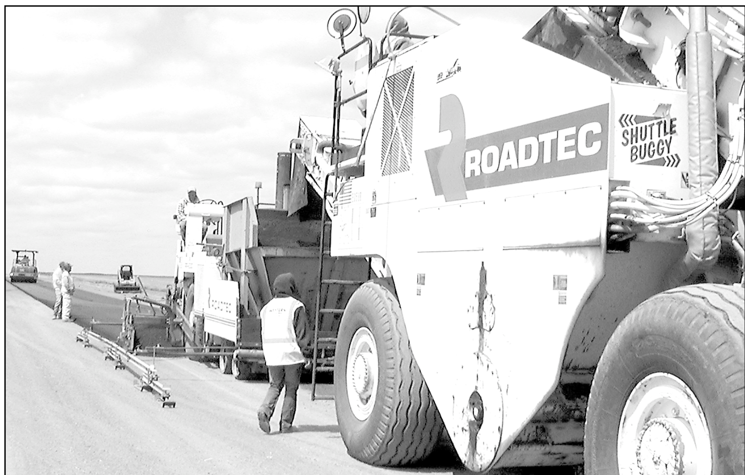
Paving is underway on the south end of the 14-mile K-27 highway project south of town, and crews from Western Engineering, the prime contractor, were near the end of the east half of the first four-mile stretch on Tuesday afternoon. A "shuttle buggy" holds about 30 tons of asphalt — about one semitrailer load — and using a conveyor belt, moves the asphalt to the laydown machine to keep an even layer of about three inches of pavement. Photo by Tom Betz/The Goodland Star-News
