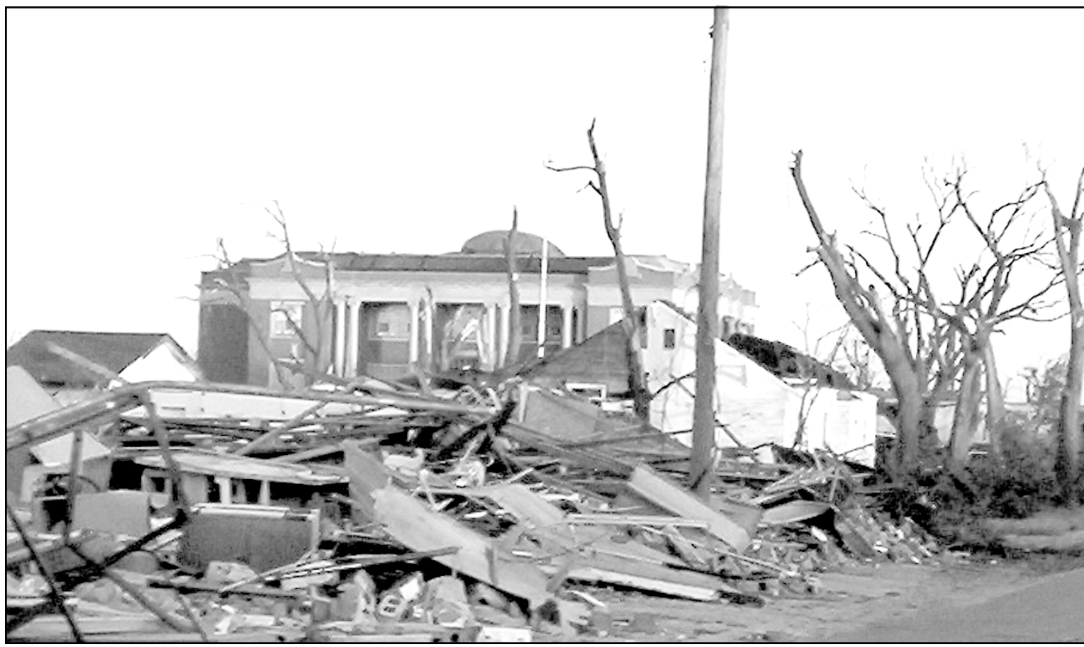
The Greensburg courthouse stands in the center of town like a beacon surrounded by devastation. Richard Breininger, who went down to Greensburg over the weekend, said it was easy to find the courthouse, the only large building standing in the town.
