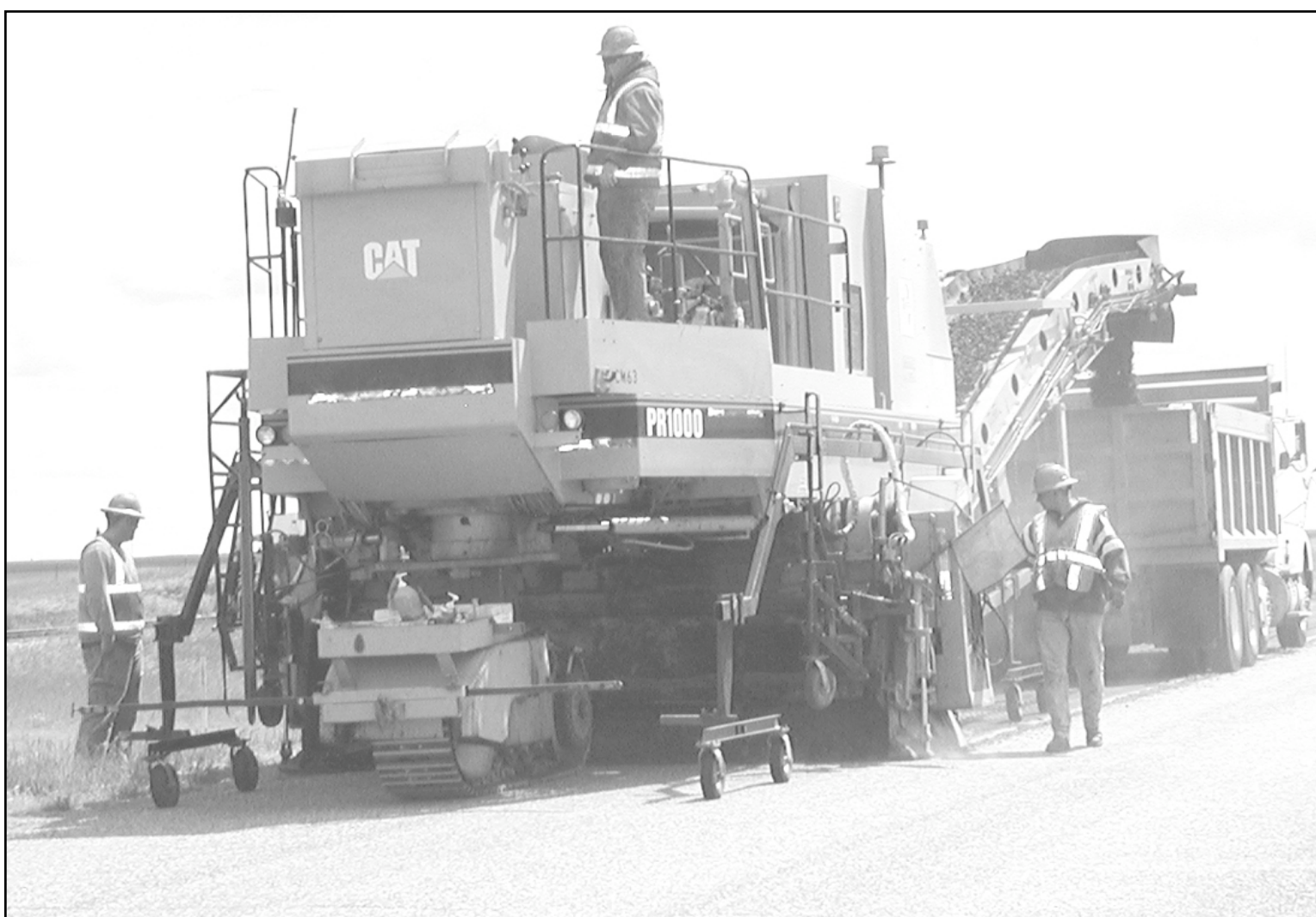
Milling work has begun on old U.S. 24 near Edson, and Wednesday a milling machine from Dustrol of Towanda was moving west of Edson milling off two-inches of asphalt. The milling machine will
