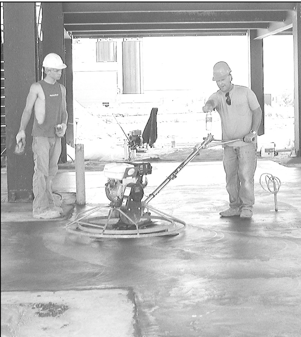
Mike Miller of Miller Construction directed a worker to a spot that needed attention as he smoothed a section of floor at the Goodland Energy Resources power plant.
