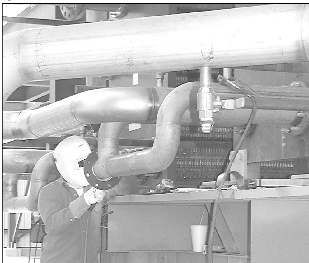
Inside the E Caruso plant a worker welded a pipe fitting as part of installing the equipment used to produce the ethanol. Construction is moving along and the plant could be producing by the end of the year.
