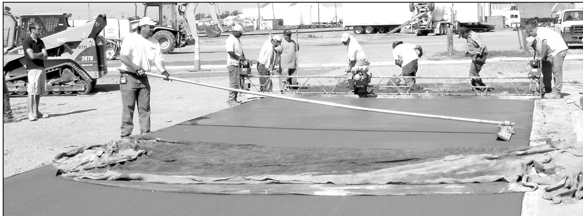
Workers from Sporer Land Development of Oakley poured the north half of the intersection at Cherry Avenue and 18th Street on Tuesday, then came back on Wednesday to pour the south half. Jerry Nemechek, engineering technician for Evans, Bierly, Hutchison and Associates, inspecting the work for the city, said the intersection should be ready after curing for a week. Nemechek said the last sections near the railroad crossing should be poured next week. Photo by Tom Betz/The Goodland Star-News
