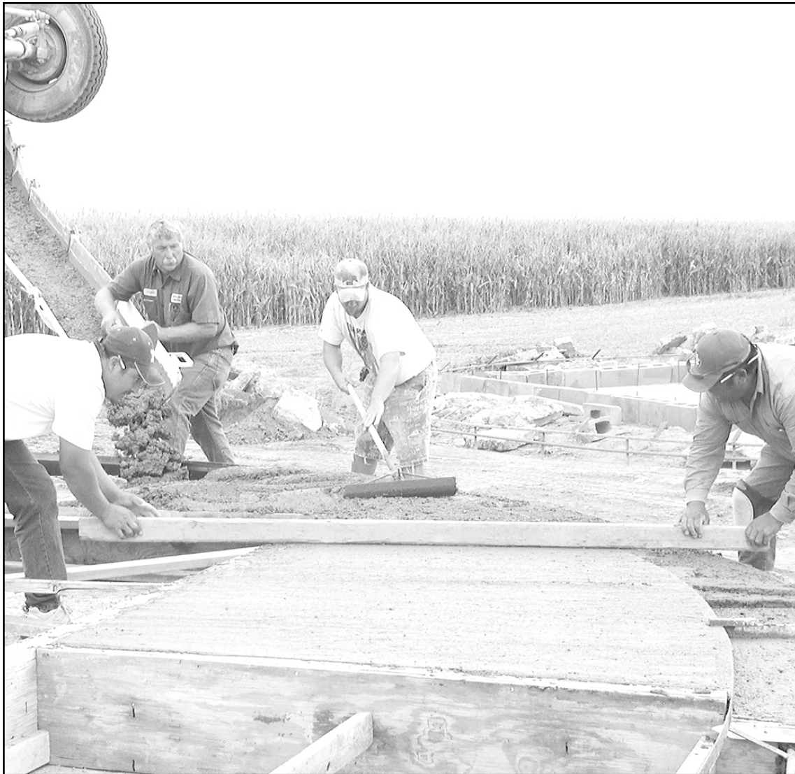
Dennis Malsom (above) scooped cement from the truck as his crew spread it out and smoothed the top at Richard Emig's farm Wednesday. Raul Hernandez (left) and his father David smoothed the surface while Ricky Koel spread cement to fill the frame of the foundation for a grain bin. Malsom (right) took several calls on his cell phone while spreading concrete.
