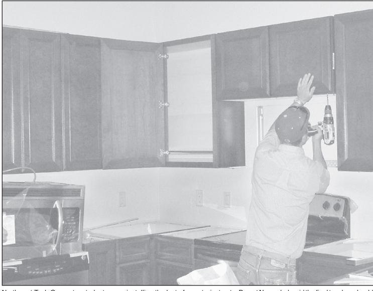
Northwest Tech Carpentry students were installing the last of the kitchen cabinets and the microwave last week as the 'green' house project is nearing completion. The kitchen counter tops were delivered earlier this week and installed on Thursday. Car-
