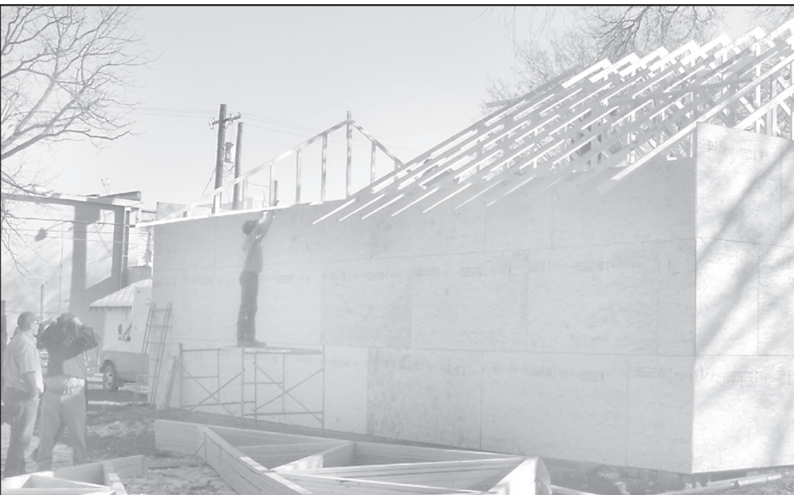
Northwest Tech students have learned a lot about remodeling an old house over the past 11 months as they rebuilt the 'green' house at 1219 Center Ave. putting on new rafters and framing the rooms inside.
