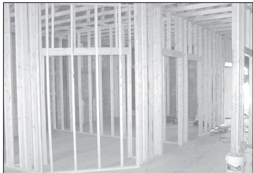
Northwest Tech students have learned a lot about remodeling an old house over the past 11 months as they rebuilt the 'green' house at 1219 Center Ave. putting on new rafters and framing the rooms inside.
