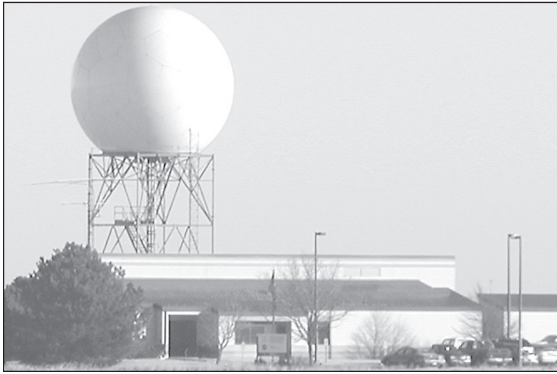
The National Weather Service radar tower is a familiar sight on the Goodland skyline. The service now has a new type of radar, Dual Polarization, which, among other things, helps distinguish different types of precipitation.
