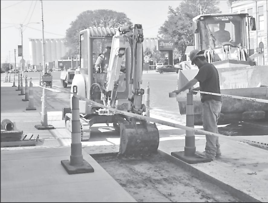
Even as the new bricks are laid between 11th and 12th Streets, work began on the sidewalks between 12th and 13th Streets. Crews have been tearing out part of the concrete in order to lay new water pipes under the sidewalk.
