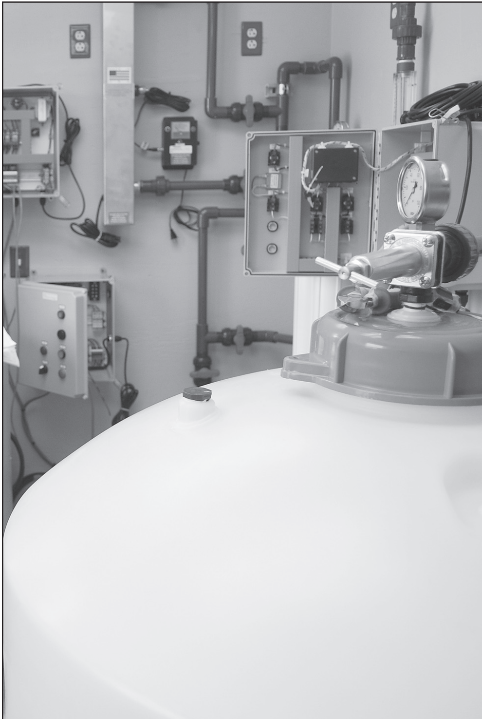
This new reverse osmosis water filtration system has been installed at Goodland Regional Medical Center specifically for the new kidney dialysis unit. The dialysis machines need heavily filtered water to operate, and the system does not connect with the rest of the hospital. – Kevin Bottrell/The Goodland Star-News
