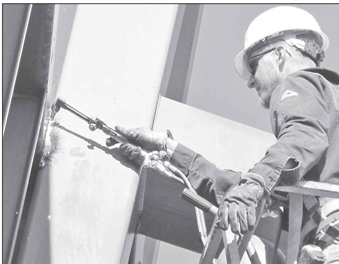
Bryant Nemechek with Nemechek Welding was responsible for cutting the welds that attach the painting to the easel. Strong welds slowed the process, but Nemechek eventually uncoupled the painting. Photos by Tom Betz/The Goodland Star-News
