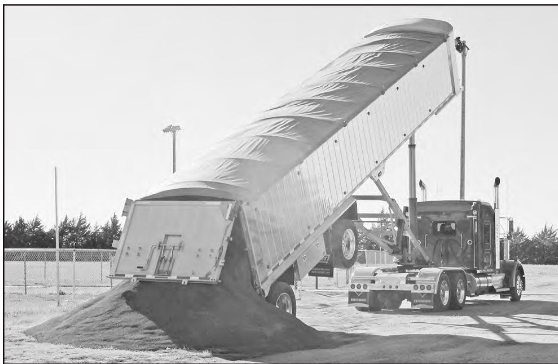
A truck dumped a load of infield conditioner at Centennial Park last week. The conditioner, which is made of clay will be applied to the infield on several softball fields.
