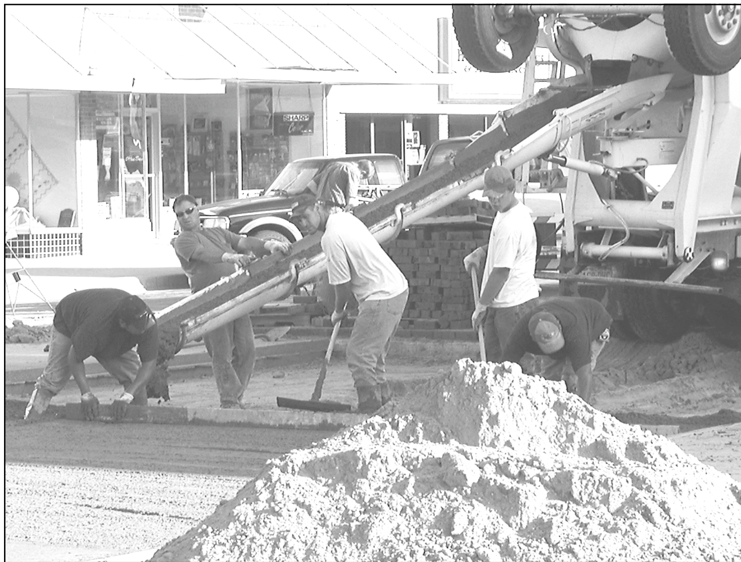
Workers from Miller Construction smoothed cement from Schlosser's Concrete at the corner of 12th and Main. The last of the cement was poured on Friday morning. The bricks will arrive in August. Photos by Pat Schiefen/The Goodland Star-News
