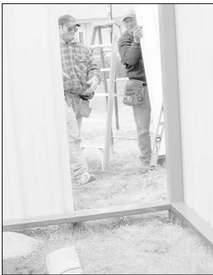
WITH CUTTERS IN HIS HAND, a worker (above) for Bainter Construction of Hoxie cut a piece of metal for the side of the carports while two men (below) put a piece of the siding up. —Herald staff photos by Kimberly Brandt
