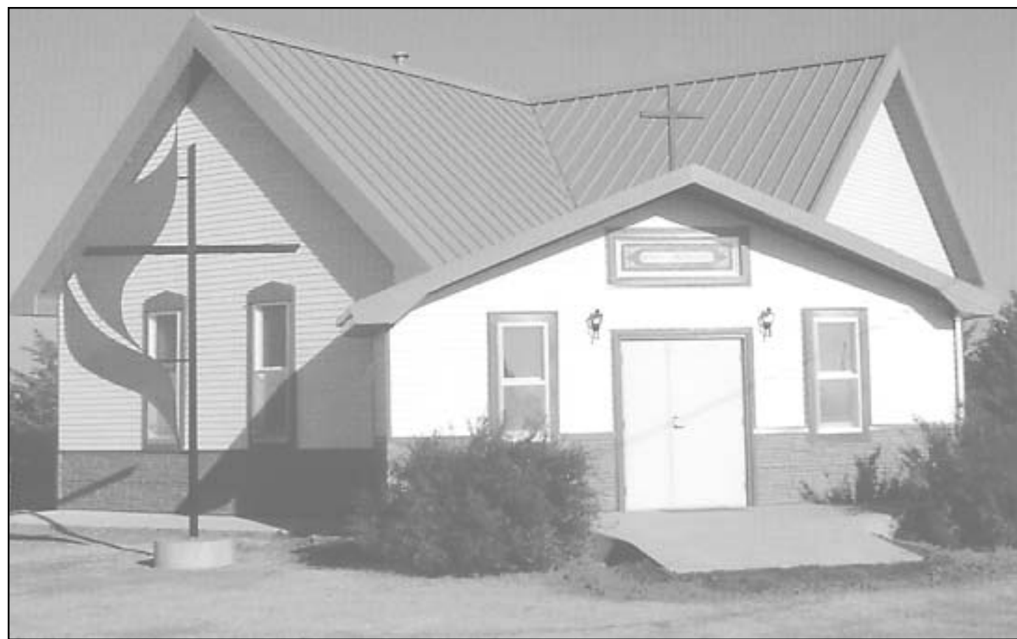
THE MCGRAW UNITED METHODIST CHURCH got a new roof (above) and white siding in August. Included in the renovations was an indoor toilet. When the church
