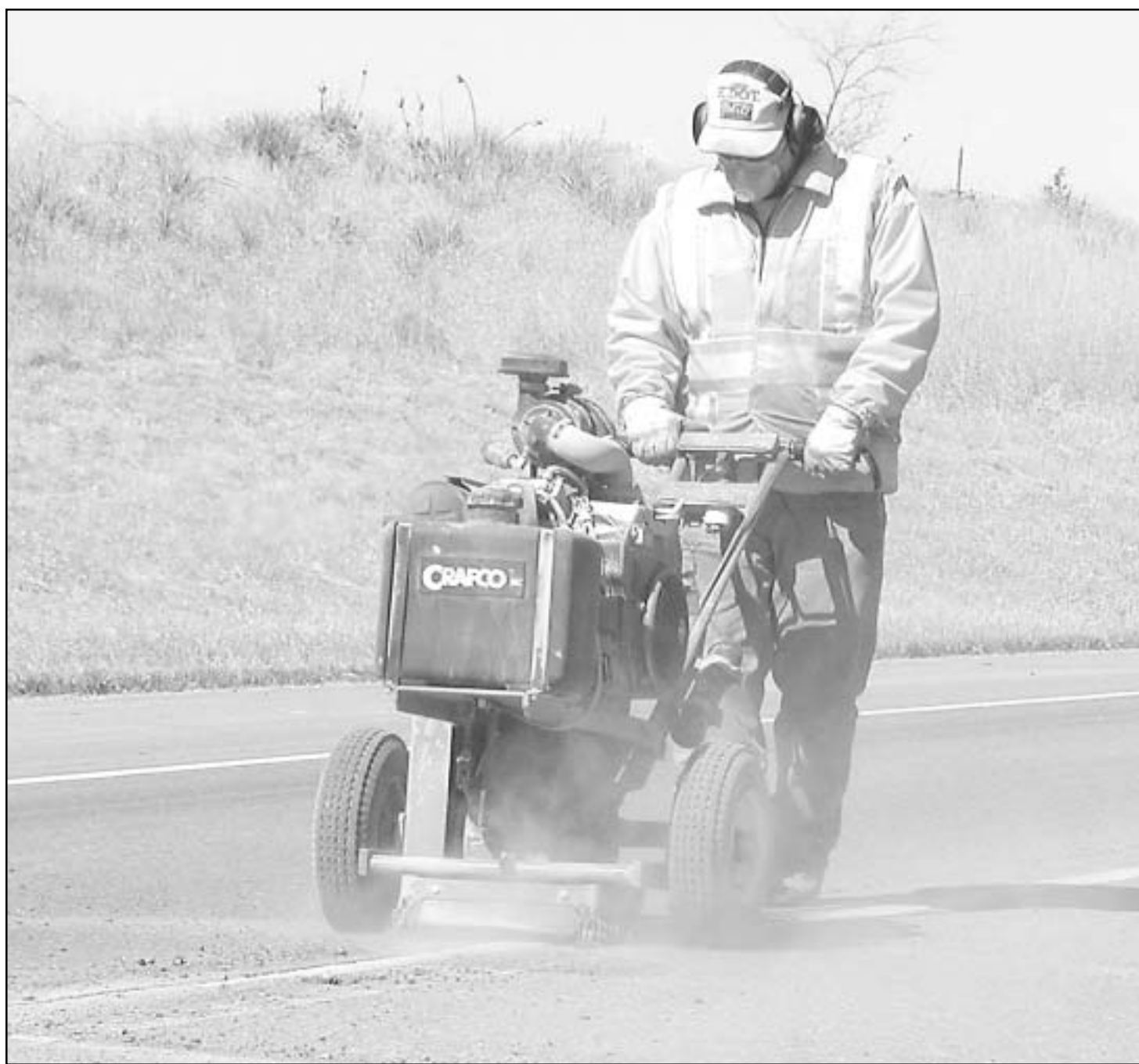
A WORK CREW from the Kansas Department of Transportation worked on U.S. 83 south of town last week. One man (above) worked with a machine to rout out the cracks
