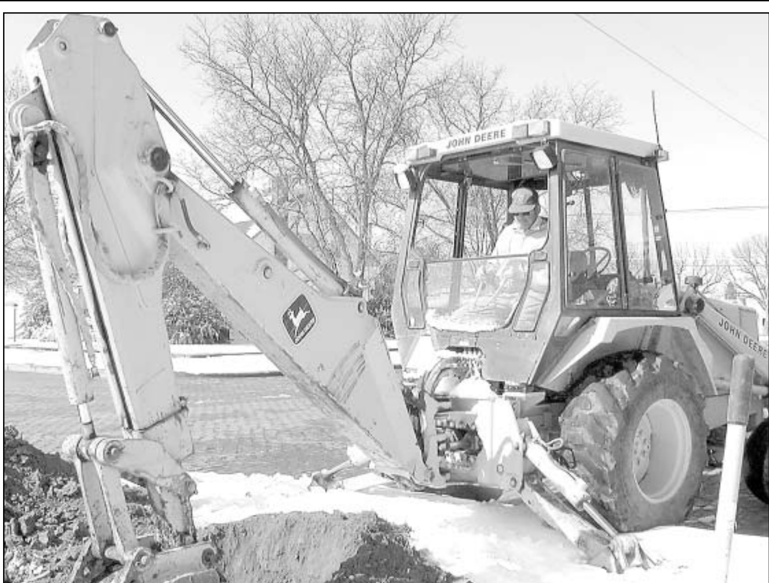
MONDAY MORNING, Willard Perrin used a back hoe to dig a hole at the intersection of Commercial and York so the city crew could replace some water valves. — Herald staff photo by Kimberly Brandt
