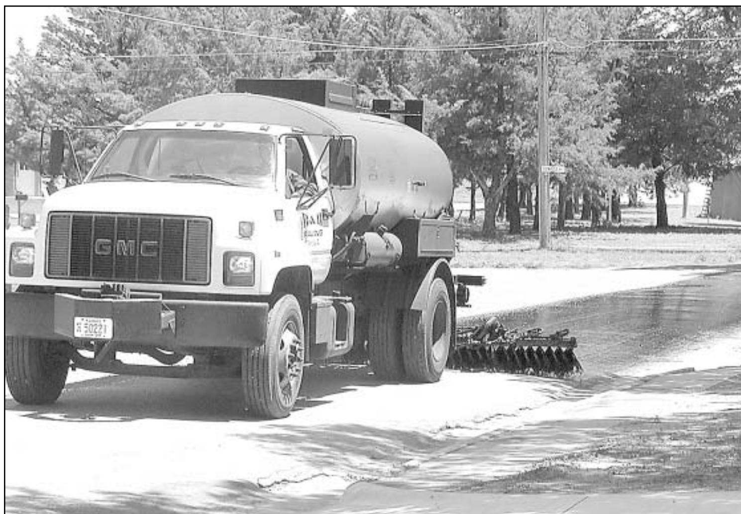
LAST WEDNESDAY , a crew with B&H Paving sprayed oil on the streets (above) with a large truck and then a machine came in and dumped sand over the oil (below). The crew did the east/west streets in town, finishing the job on Thursday.
