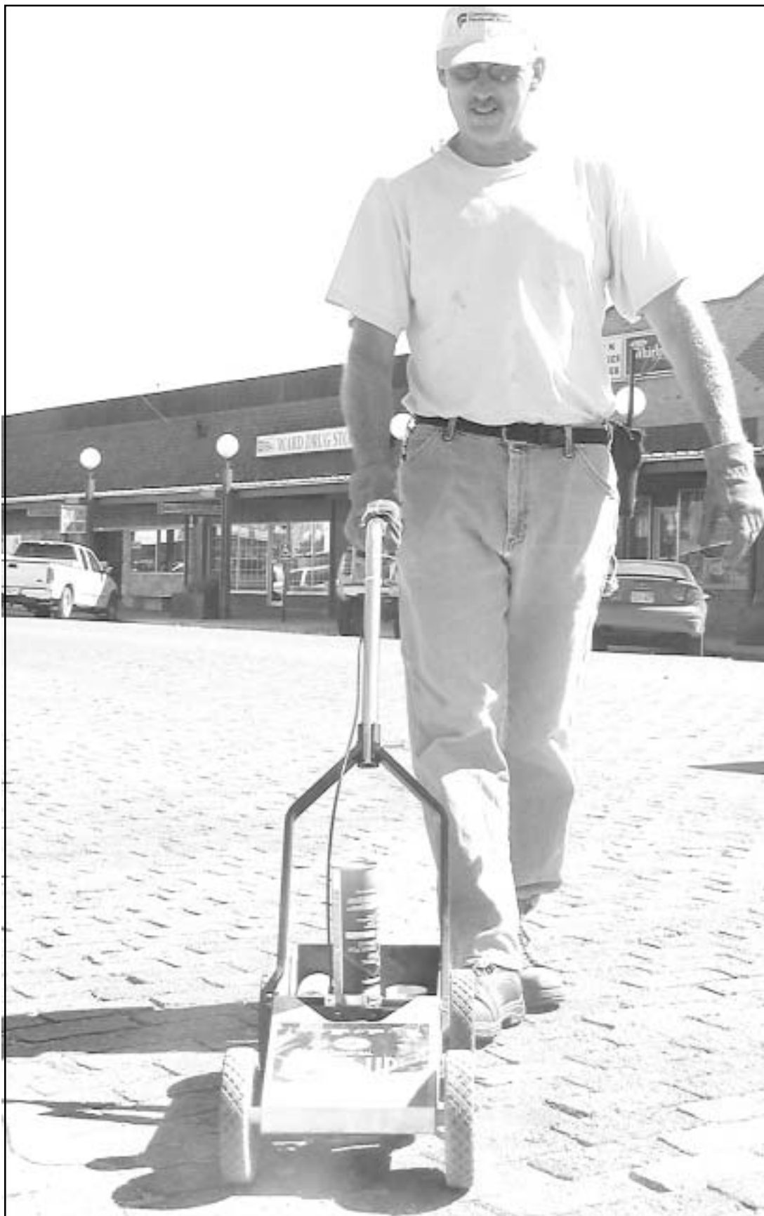
PUSHING A SPRAYER, City employee Bob Shuler was busy painting yellow parking lines on the brick streets in downtown Oberlin on Monday. The little paint machine had no guides, he said, so he was just hoping for straight lines, and it required several passes to get a thick enough line.
