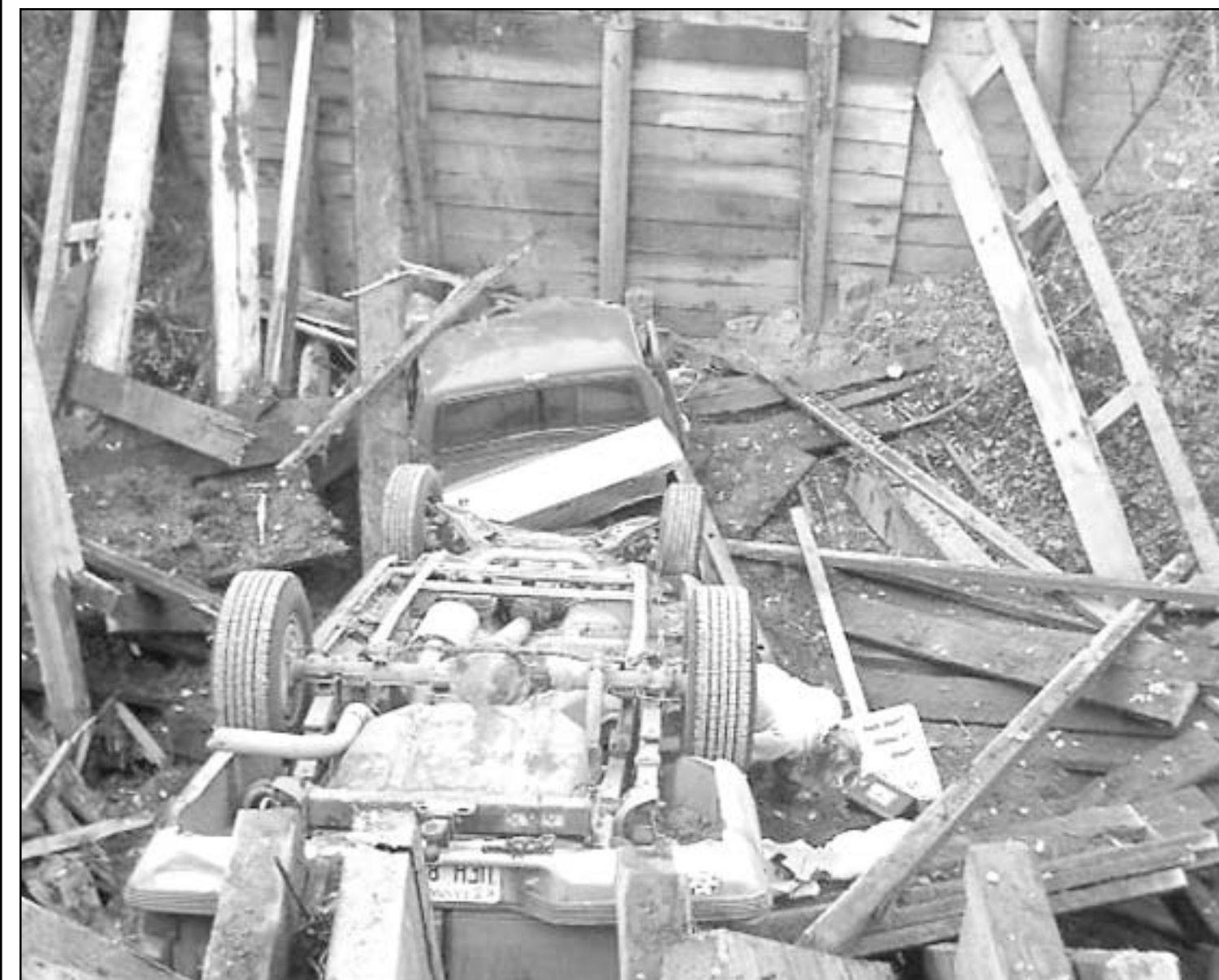
TWO VEHICLES (above) wound up in the creek bed north of Norcat on Thursday night after the drivers tried to cross a bridge that had collapsed. The pickup landed on its wheels and the Suburban landed upside down in the box of the truck.
