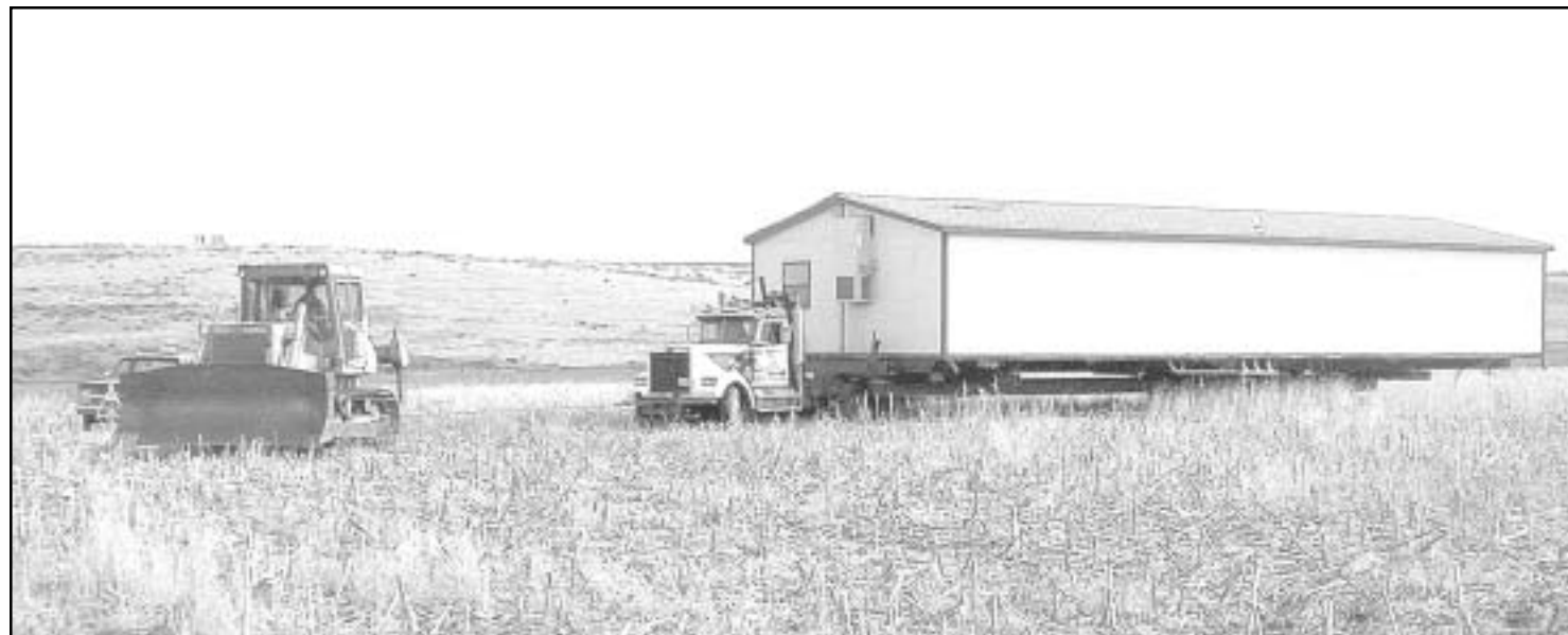
FRIDAY AFTERNOON , a county road dozer (above) helped pull a semi-trailer truck loaded with a 28x60-foot modular classroom across a corn field belonging to Lee
