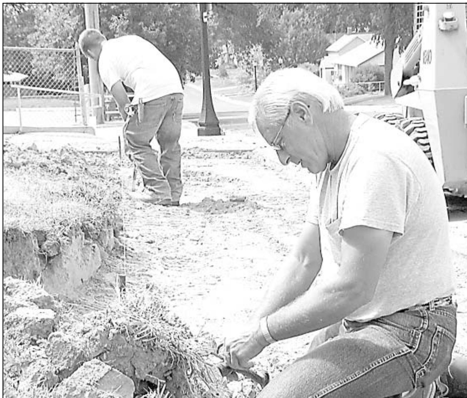
OUTSIDE THE GRADE SCHOOL Monday, Ron Beneda, head lineman with the city crew, fixed an electrical line hit by a crew putting in a sidewalk on Cass Avenue near the kindergarten building. — Herald staff photo by Kim Davis
