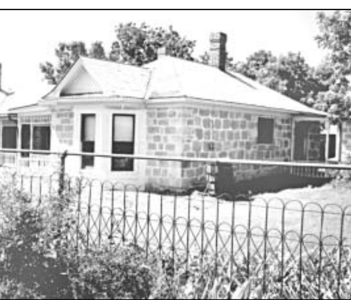
THIS STONE HOUSE (above) was the home built by Fenton Pratt in the 1880s and 1890s. It still stands, along with four other original stone buildings at the Cottonwood Ranch, a half mile west of Studley.
