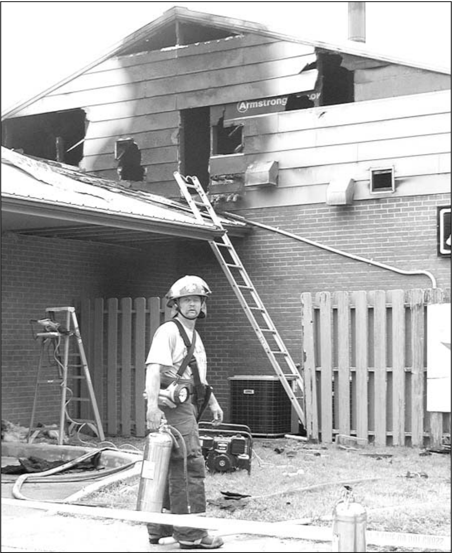
AT CENTENNIAL BOWL, Fireman Randy Peters (above) got ready to cool off the hot roof after a blaze destroyed the building. Gary Zodrow (below) pulled supplies
